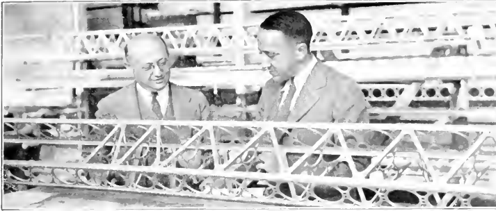
Dr. Karl Arnstein, vice-president and director of engineering for The Goodyear-Zeppelin Corporation, inspecting, with an assistant, built-up Duralumin struts for the frame for the Akron (ZRS-4). (Dr. Arnstein is at the left in the photograph).
